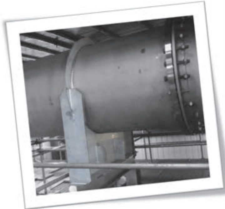
Example of a Stainless Steel Large Bore Saddle designed & manufactured by QPS
